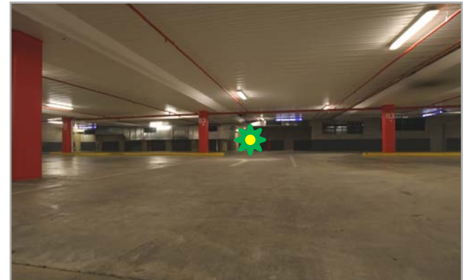
View of Carpark "Level -3"
